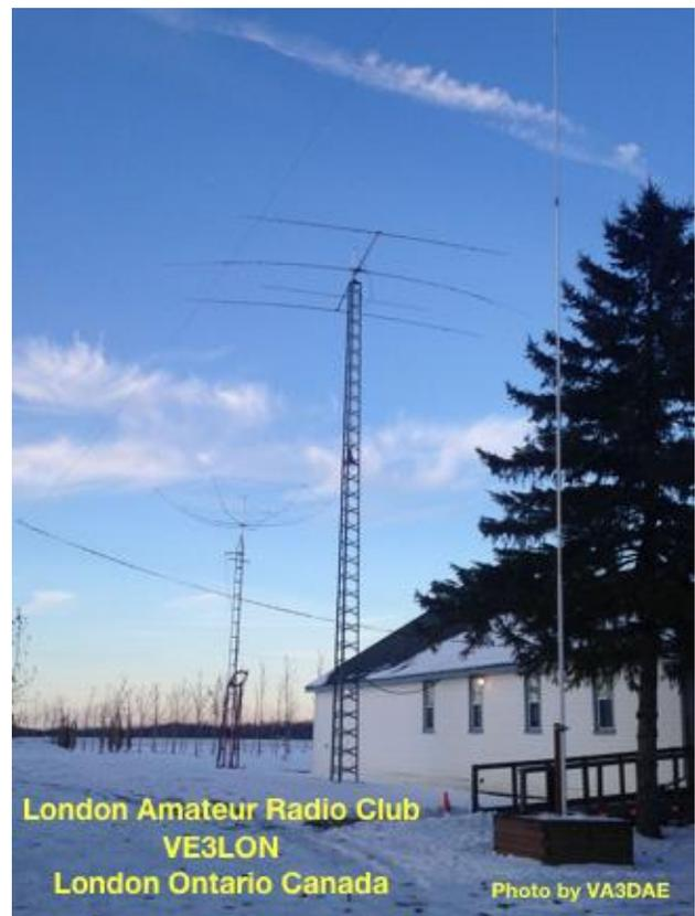
*QSL card for LARC club station VE3LON showing the Yagi, Hex-Beam, Vertical, and Dipole antennas.*
